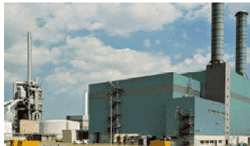
Gas-fired power generation
